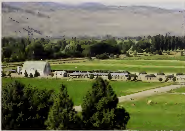
Livestock handling facility at Kamloops
