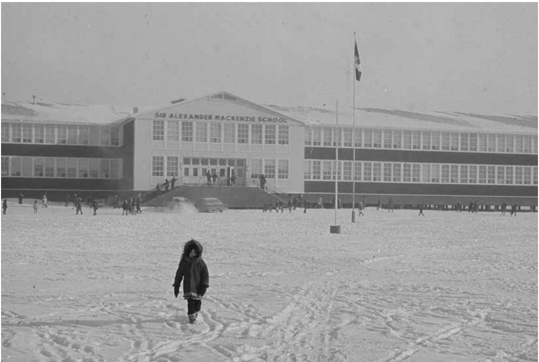
The exterior of Sir Alexander Mackenzie School in Inuvik, Northwest Territories, April 1970. The school had two separate wings: one Catholic, one Protestant. Public Works and Services, Northwest Territories Archives, Wilkinson/N-1979-051: 0409S.
