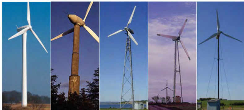
Tubular steel tower
